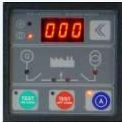
load and generator, feeding the load from either Mains or Generator bus-bars, whichever is available, with mains bus-bar priority.
